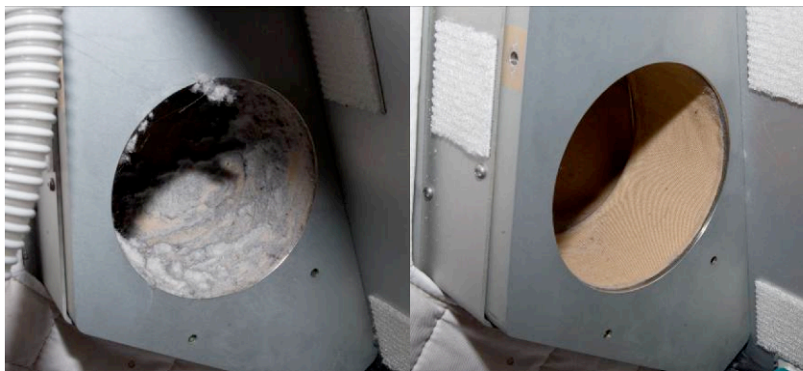
Figure 5. Starboard CQ intake duct (pre- and post-cleaning).
