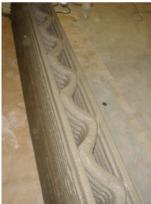
Figure 17: Contour Crafting concrete printing of walls and other elements, nozzle (left), printed concrete wall (right), courtesy of the Center for Rapid Automated Fabrication Technologies (CRAFT) at USC
