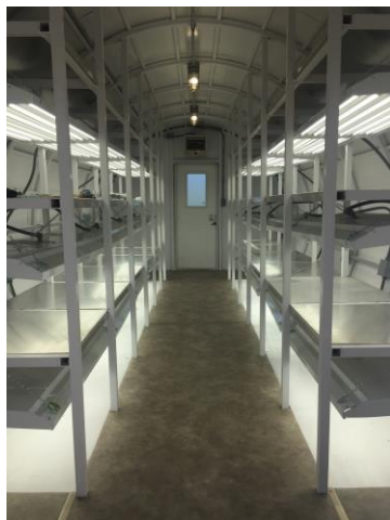
Figure 21. Plant Production Module. Adjustable lights emit wavelengths conducive to plant growth.
