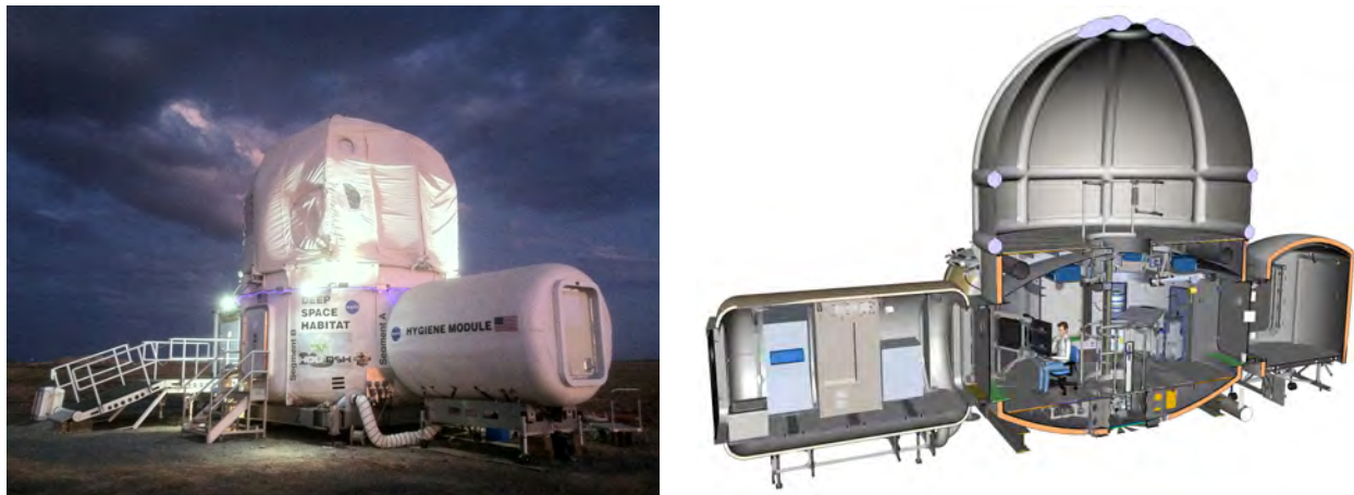
Figure 1: Habitat Demonstration Unit, 2011 D-RATS configuration with U. Wisconsin X-Loft (left), section (right)
