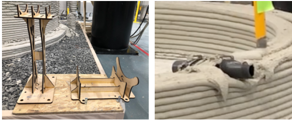
Fig. #17. (Left) Bases for pipes. (Right) Avoidance of pipe by the printhead after emplacement
