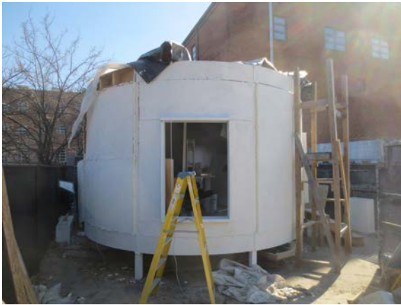
Figure 4. Exterior of HAVEN habitat under construction
