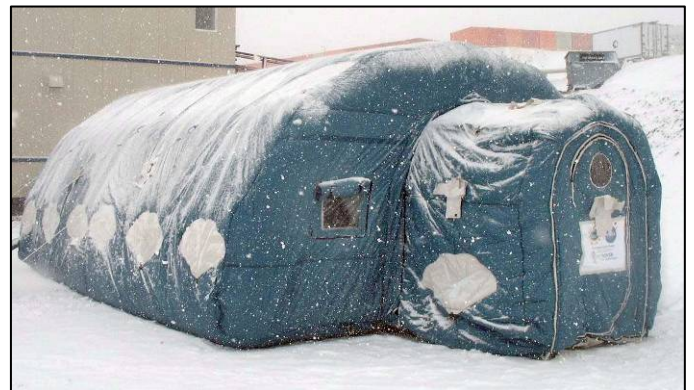
Figure 8 – Airlock, Door and Window Details
