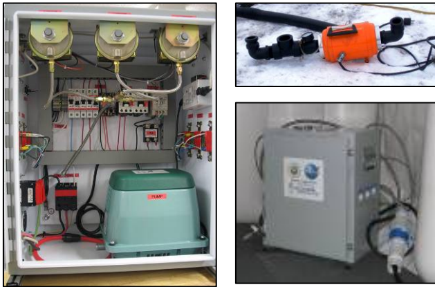
Figure 11 – Inflation System Components - Internal Make-up Pump & Power Distribution System Door open & Closed and Orange External Inflation Blower
