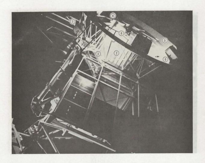
Transfer Worksite Support Equipment: (1) Primary Foot Restraints; (2) Transfer Workstation Light; (3) Dual Translation Rails; (4) Sun End Primary Cargo Stowage Receptacle; (5) Sun End Cargo Temporary Stowage; and (6) Sun End Workstation Lights.
